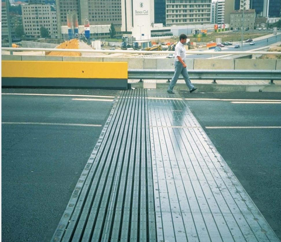
*Algaflex TM is the last development of a highly tested technology by Alga in the field of medium and big movement joints.*
